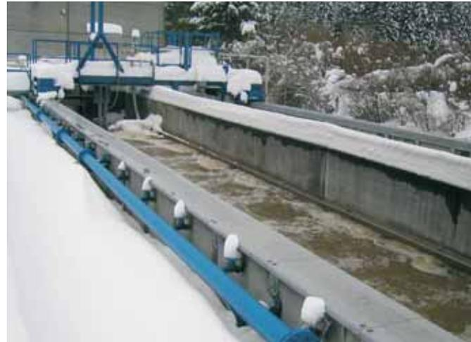
operating prototype plants which are kept ice-free by the intelligent change of scraper design only.
